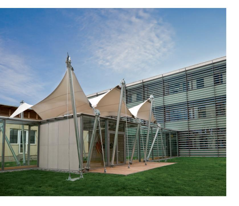
The corridor connecting the existing infrastructure with the new building. Underneath the terrain, orthogonally to the above-ground part of the new building, are located clean room laboratories.
